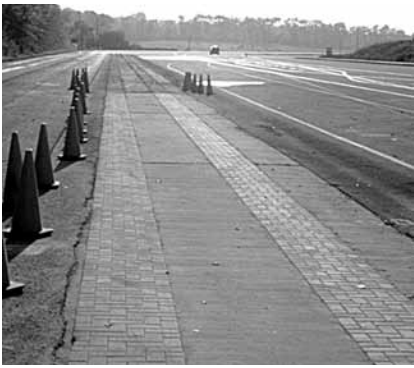
Figure 5. The test track section and concrete paver surface at The Pennsylvania Transportation Institute test facility.
