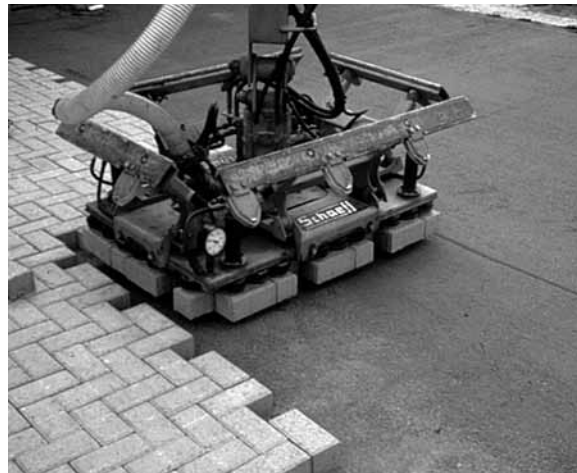
Figure 6. The vacuum head over the paver layer.
