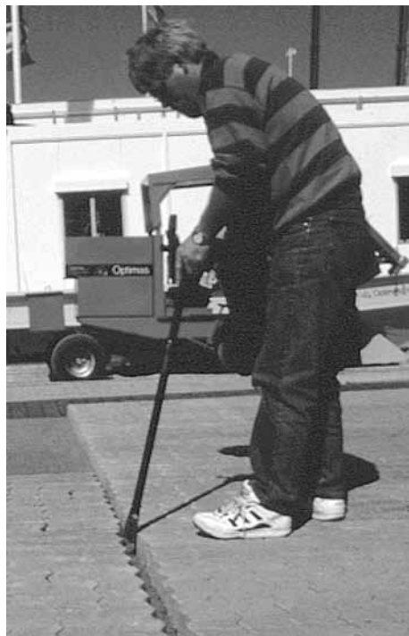
Figure 21. Once a few layers are removed by hand, then adjacent layers can be separated with a pry bar.
