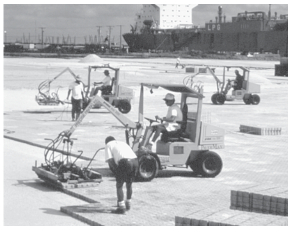
Figure 1. Mechanical installation equipment at Port of Tampa, Florida.
