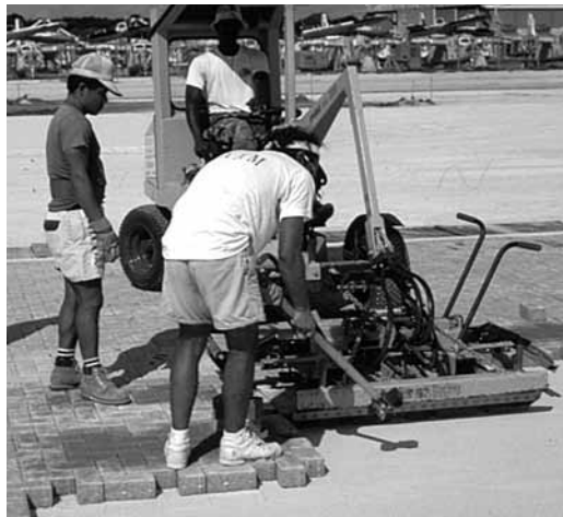
Figure 5. Motorized equipment with a hydraulic clamp.
