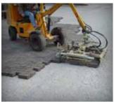
Mechanical installation equipment accelerates construction; typical 5,000 sf (500 m²)/machine/day. After placement, joints and/or openings filled with small aggregate and pavers are compacted.
