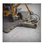
Aggregate base is spread and compacted; pavers are delivered ready to install. After placement of bedding course, joints and/or openings are filled with small aggregate and the pavers are compacted. Joints may be filled mechanically as shown. Mechanical installation speeds construction. Base construction uses locally available materials.
