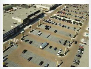
350,000 sf (3.2 ha) of PICP at a Burnaby, BC shopping center infiltrates runoff from roofs.
