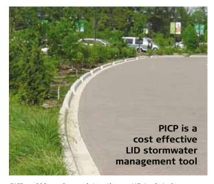
PICP and bioswales work together as LID tools to increase infiltration at Morton Arboretum in Lisle, IL.
