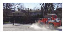
Mechanical sweeping of fine aggregate into paver joints
