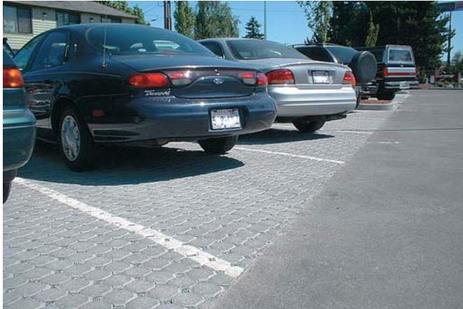
Ash Avenue Park and Ride - Marysville, WA
