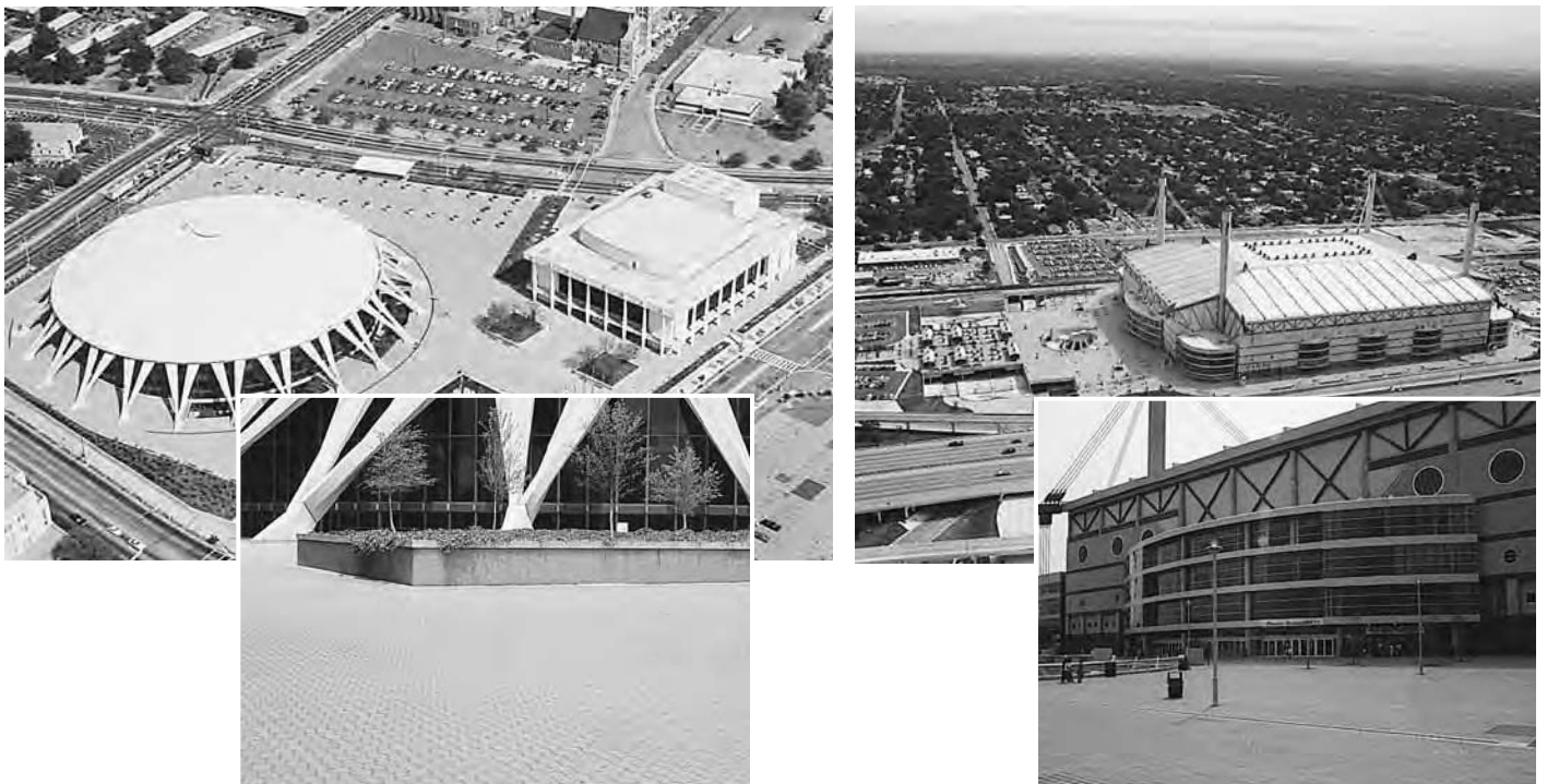
Figure 21. The plaza area around Scope Center in Norfolk, Virginia, (left) and one side of the Alamo Dome (right) in San Antonio, Texas, include roof plaza decks surfaced with concrete pavers.
