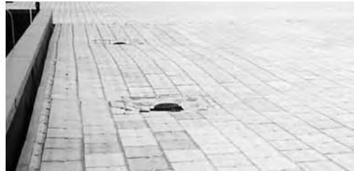
Figure 4. Some ballast-type slabs for roof decks are made with lightweight concrete materials. They can be joined with tongue-and-grooves and/or with connectors to resist wind uplift. This is one of several designs available.
