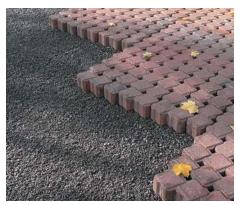
Ecoloc<sup>®</sup> pavers were placed on a bedding layer of ODOT 02610.10 open-graded aggregate
