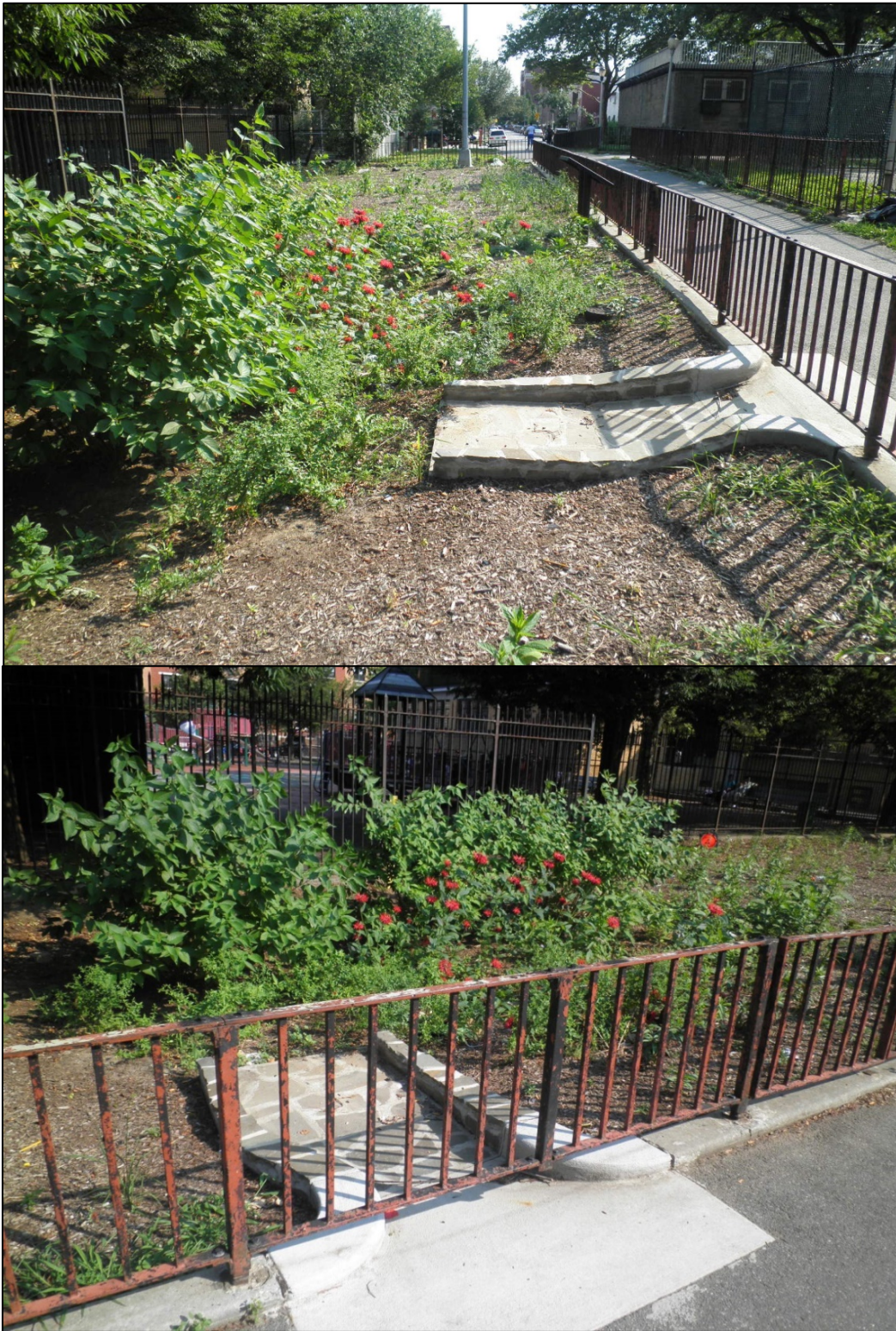
Figure 3-22: On-site Bioretention in Demo Area 3 Showing Curb Cuts and Plantings
