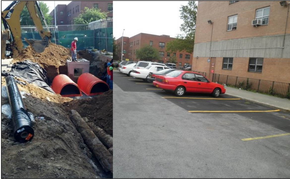
Figure 3-23: Demo Area 3 Subsurface Detention System During and After Construction
