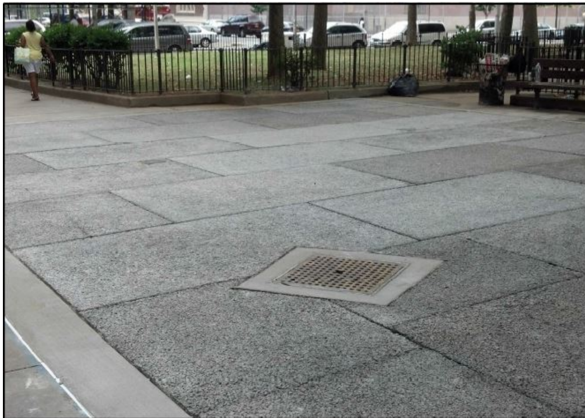
Figure 3-14: Demo Area 2 Porous Concrete Panels and Inlet Grate at NYCHA’s Seth Low Houses
