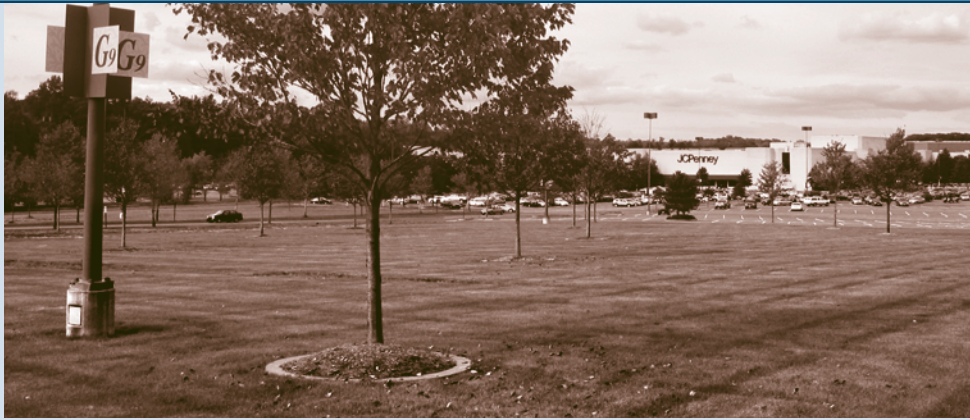
One solution to the problem of too much parking: Westfarms Mall in West Hartford and Farmington features an engineered grass overflow parking lot, to promote infiltration of stormwater.
