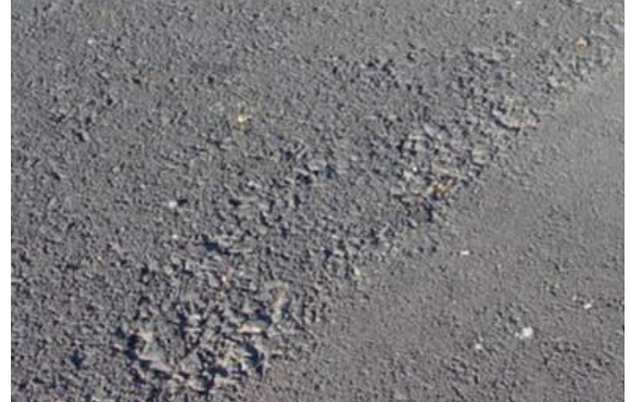
Figure 4-5. Pervious asphalt in Raleigh, North Carolina
