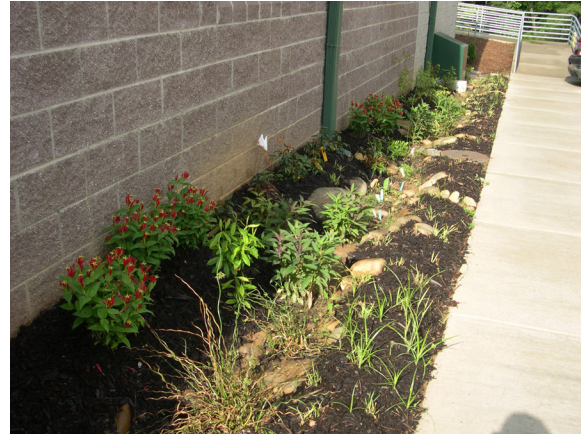
Figure 8-23. Water discharged from the green roof is released to this linear rain garden at the Operations Center
