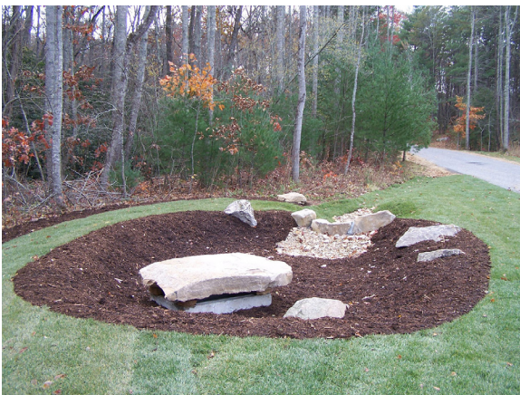
Figure 8-8. Bioretention cell after construction (courtesy of David Tuch, Equinox Environmental)
