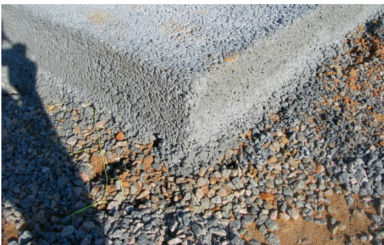
Figure 4-4. Pervious concrete in Nashville, North Carolina
