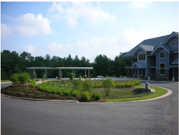
Figure 8-27. Baker Center rain garden at the North Carolina Arboretum just after initial planting
