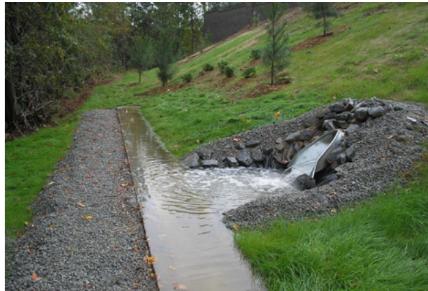
Figure 4-13. Metal level spreader in Apex, North Carolina
