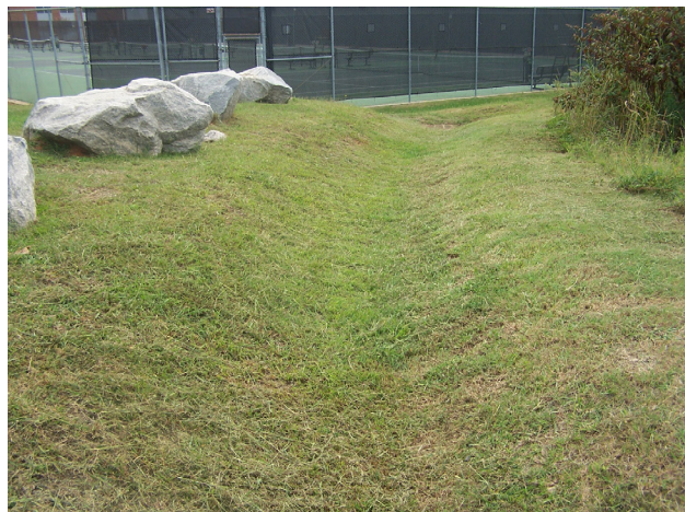
Figure 4-9. Dry swale in Raleigh, North Carolina
