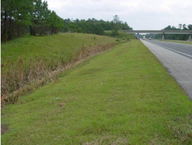
Figure 4-10. Wet swale along I-40 in eastern North Carolina
