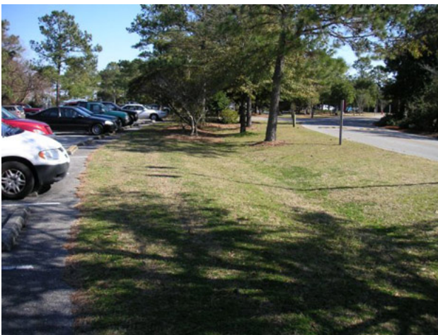
Figure 3-11. Disconnected impervious surfaces
