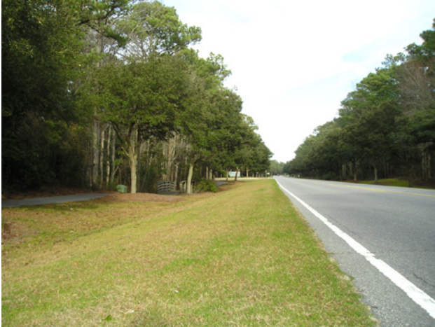
Figure 3-2. Vegetated areas combined with roadways
