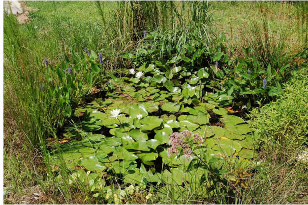
Figure 4-8. Pocket wetland serving a watershed smaller than one acre
