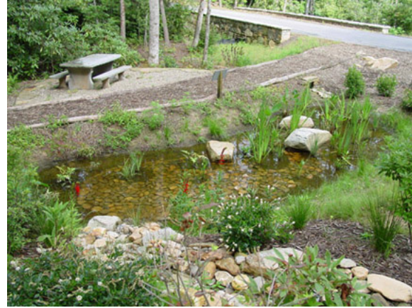
Figure 8-9. Stormwater wetland (courtesy of David Tuch, Equinox Environmental)
