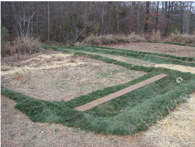
Figure 4-12. Concrete level spreader in Apex, North Carolina
