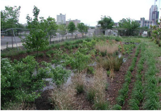
Figure 4-2. An ultra-urban bioretention cell in Charlotte, North Carolina
