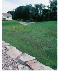
Stormwater runoff from the traditional section is collected by curbs and catch basins, then piped through a stormwater treatment system. The BMP neighborhood utilizes a number of structural and non-structural practices including grass swales, vegetated bio-retention areas, roof leader rain gardens, "low-mow" zones, street sweeping, fertilizer and pesticide management, and
