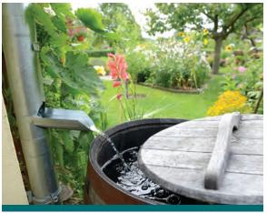
**Figure 3.5.1:** Rainwater storage tanks can hold more water than rain barrels and can be installed outdoors above ground for seasonal use, or buried below ground for year-round use.
