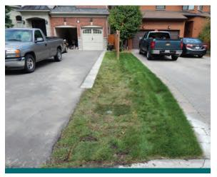
**Figure 3.4.3:** This photo shows the infiltration trench shortly after the turf installation. Instead of turf, plantings could have been incorporated into the design. (Source: Aquafor Beech)
