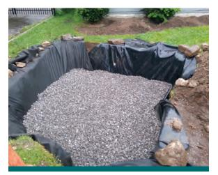
**Figure 3.4.1:** Construction of a residential soakaway. (Source: CVC)
