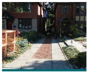
Figure 3.3.2: A strip of pervious gravel with large block pavers. (Source: Aquafor Beech)
