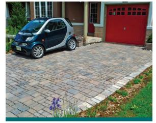
**Figure 3.3.1:** A driveway paved with permeable interlocking pavers. (Source: Fern Ridge Landscaping)
