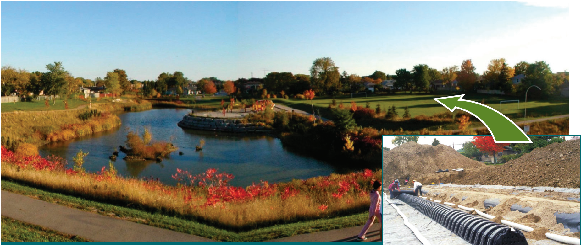
Figure 3.1.5: A combined integration strategy was used at Terraview Park in Toronto. Some stormwater features enhance the aesthetic value of the park, while an infiltration chamber was installed below a soccer field to treat water from a 40 hectare area. (Source: Aquafor Beech)
