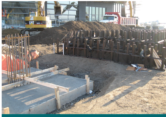
Figure 8.4.1: Proper installation of soil support systems ensures settling does not occur and maintenance is not required. (Source: Deep Root)
