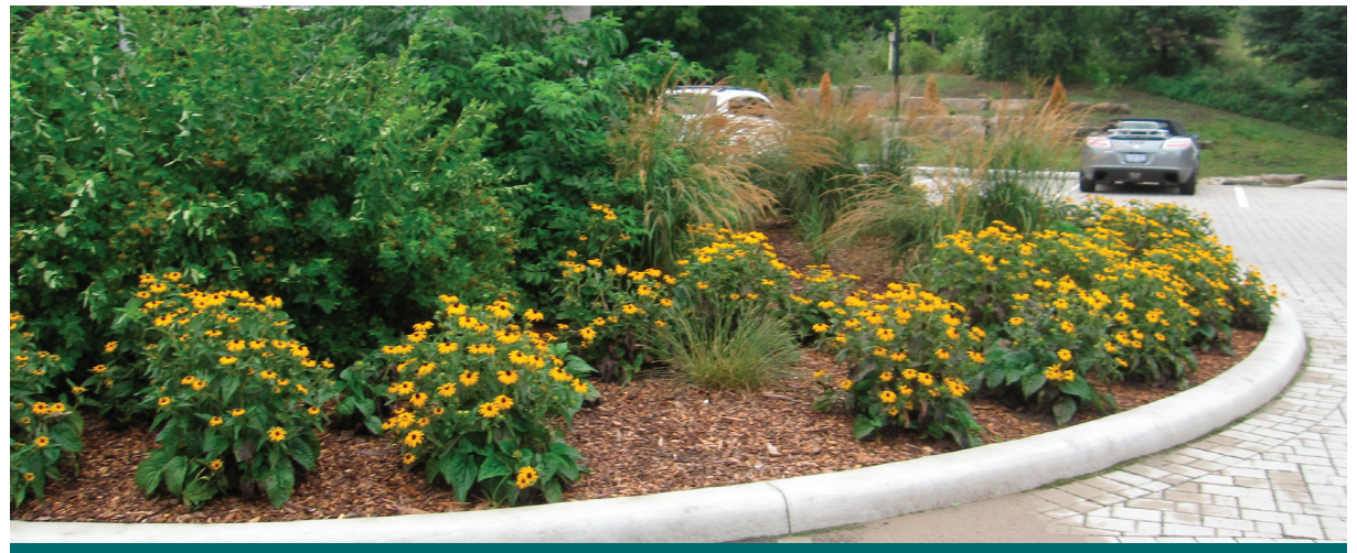
Figure 2.1.1: This bioretention facility at Kortright Center for Conservation has a beautiful aesthetic and is surrounded by curbs which provide a protective barrier from vehicles. (Source: CVC)
