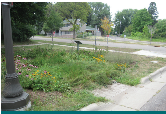
Figure 3.3.2: Urban parkettes may look small, but they have the potential to treat a large surface area of road. Typical ratios of impervious drainage area to bioretention range from 5:1 to 15:1. (Source: CVC)
