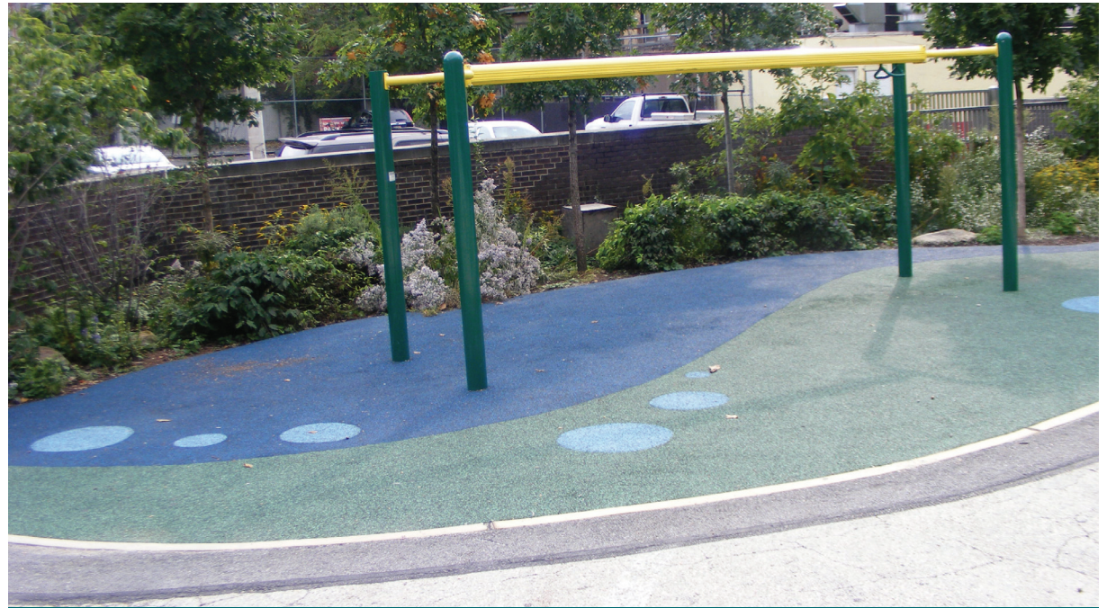
Figure 3.0.1: It is essential to hold public consultations when retrofitting active areas to ensure that user needs are fully understood and met. This playground incorporates both bioretention and a permeable bonded rubber as a user-friendly alternative to permeable pavers. (Source: Aquafor Beech)
