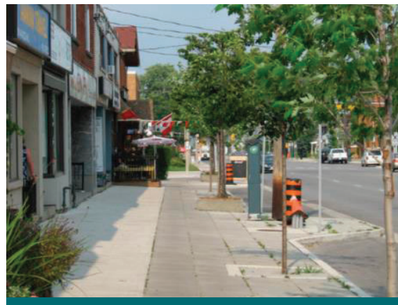
Figure 2.6.3: Sidewalk after construction with healthy trees. (Source: Deep Root Inc.)
