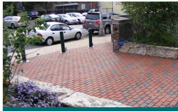
Figure 2.3.3: Coloured pavers can be arranged in patterns in public meeting spaces like this urban park. As part of a water balance based stormwater management strategy, permeable pavers can help alleviate urban flooding during intense rainfall events. (Source: Aquafor Beech)
