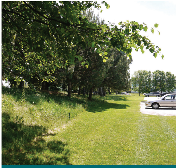
Figure 4.4.1: A no-mow zone is a small-scale LID retrofit option. (Source: Aquafor Beech)
