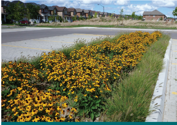
Figure 3.3.1: The bioretention area installed at O'Connor Park in Mississauga is part of a stormwater management system that treats parking lot runoff prior to discharging to a local wetland. (Source: CVC)
