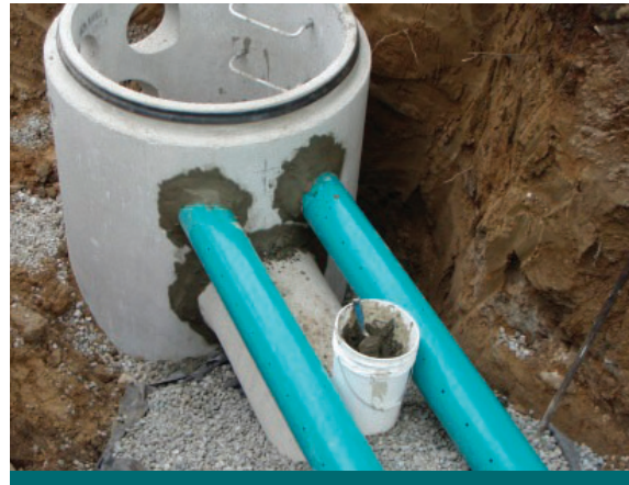
Figure 2.5.1: Perforated pipe systems use many of the same materials and construction practices as conventional storm sewer pipes while also encouraging infiltration. (Source: Aquafor Beech)
