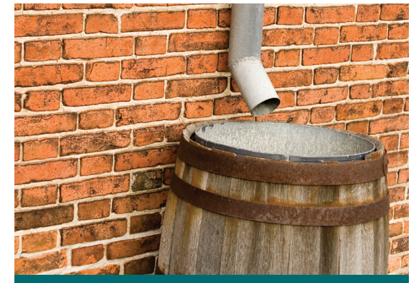
Figure 5.1.1: Rain barrels are a simple retrofit option for roofs with exterior downspouts.
