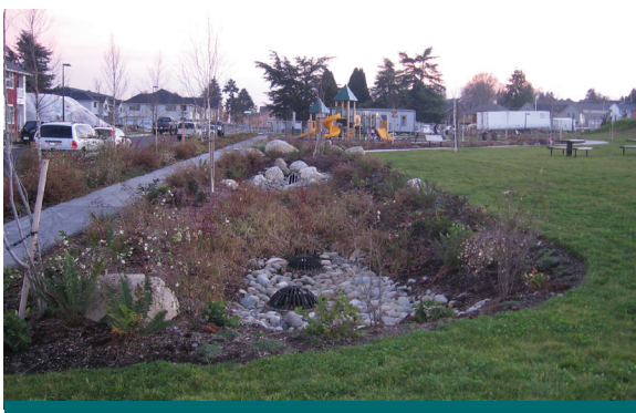
Figure 3.3.3: The road surface (left) contributes significantly more stormwater pollutants than the parkland area (right). To achieve maximum watershed benefit a designer could consider accepting runoff from this external area. (Source: CVC)
