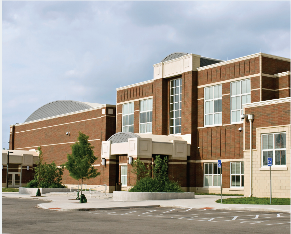
Figure 1.6.1: There are many different options for retrofitting school grounds. Rainwater harvesting, green roofs or parking lot bioretention are just some of the ways you can better manage rainwater on your property.
