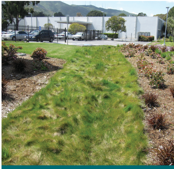
Figure 2.2.1: This enhanced grass swale uses a low maintenance fescue grass which only needs to be mowed once or twice a year. The taller grass provides added filtering and enhanced texture. (Source: CVC)
