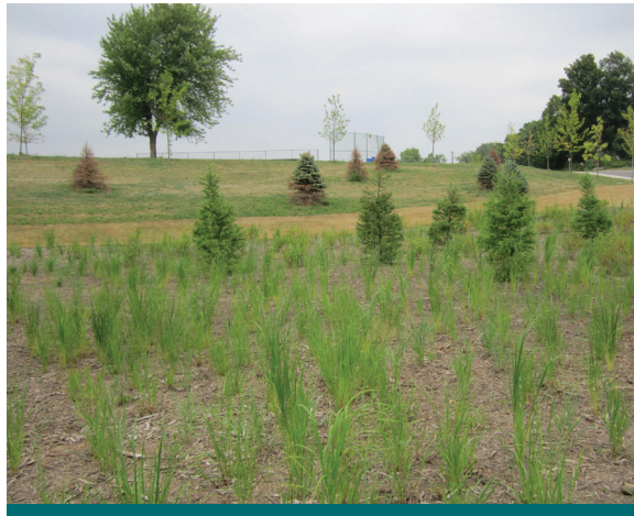
Figure 3.1.3: To reduce localized flooding, consider this practice in areas that are prone to ponding water. This bioretention practice was installed in a low-lying area. (Source: LSRCA)
