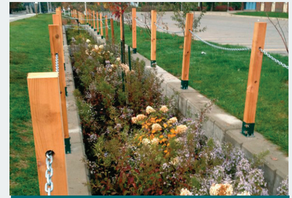
Figure 1.6.2: Elm Drive is a project involving Peel District School Board and City of Mississauga. This project replaced aging ditches with bioretention planters and improved street parking in front of the school. (Source: CVC)
