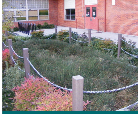
Figure 5.3.2: This bioretention practice accepts drainage from adjacent hard surfaces and provides stormwater controls. Posts and chains are provided to prevent damage from foot traffic. (Source: CVC)
