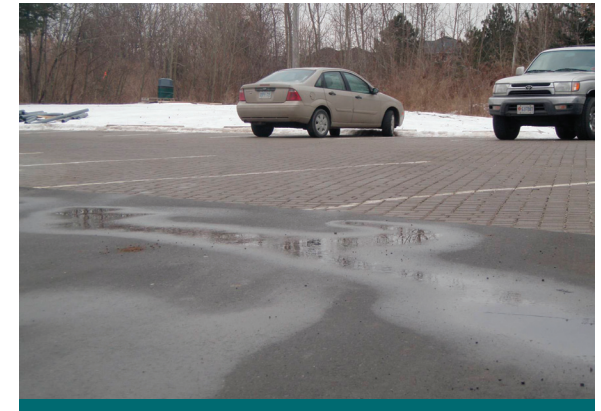
Figure 4.1.3: Installing permeable pavement in your parking lot may reduce the quantity of de-icing salt used on your site. Permeable pavement provides good traction for pedestrians and prevents ice formation by providing quick drainage to the granular layer below the pavement surface. Reduced risk of slips, trips, and falls is a strong retrofit incentive. (Source: CVC)
