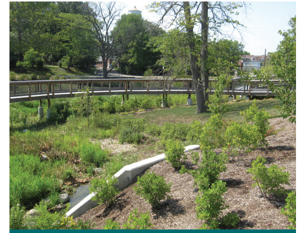
Figure 3.1.4: A boardwalk gives pedestrians a complete view of this bioretention practice. The pathway also prevents damage to the facility from foot traffic. (Source: CVC)
