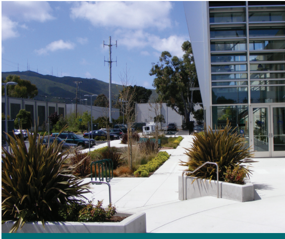
Figure 4.3.3: Bioretention planters beautify this building entrance. The entrance receives a lot of traffic during business hours, making it an ideal location for a high visibility LID practice. (Source: Aquafor Beech)
