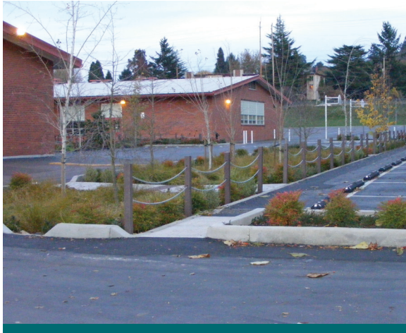
Figure 5.3.1: At this school property, bioretention is contained within parking lot islands. Note the sidewalks that have been included for pedestrian flow. (Source: CVC)
