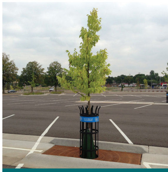
Figure 2.6.1: Precast tree planters can be used independently or as part of a treatment train with other LIDs. (Source: CVC)
