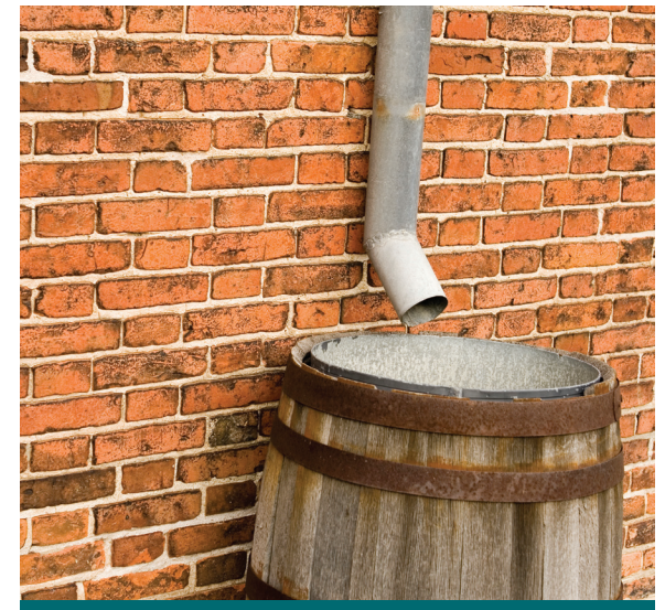
Figure 7.1.2: A rain barrels is a simple retrofit option that does not require extensive effort to implement.
