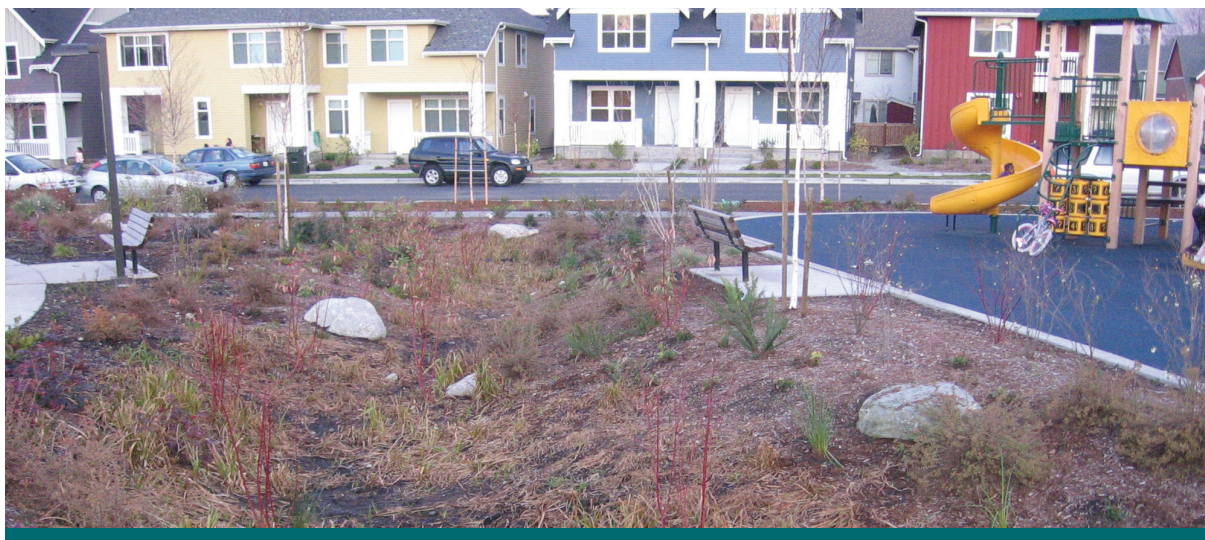
Figure 3.4.2: When installing new parks equipment, consider whether the LID practices can be integrated into the design. Here a bioswale has been built into the landscape between a playground and sidewalk. (Source: CVC)
