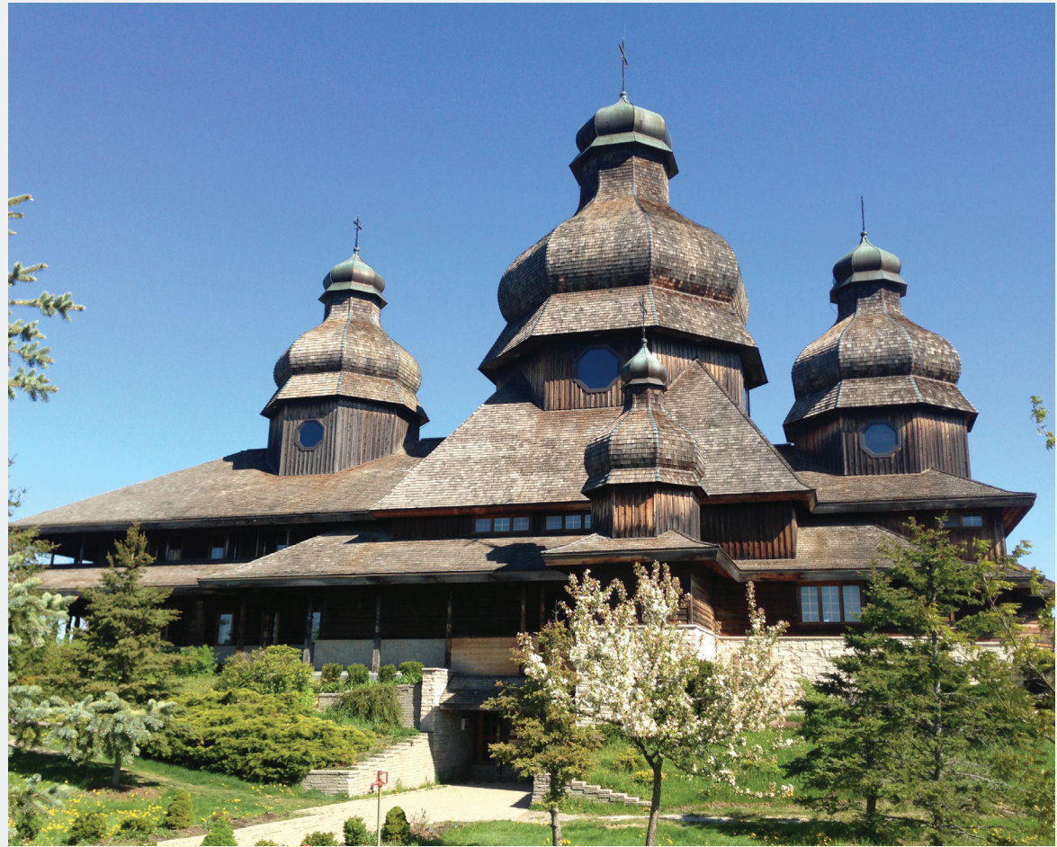
Figure 1.8.1: LID retrofits are ideally suited to addressing issues with drainage. Rain gardens or bioswales could be installed along this path, intercepting rainwater before it ponds at this basement entrance.
