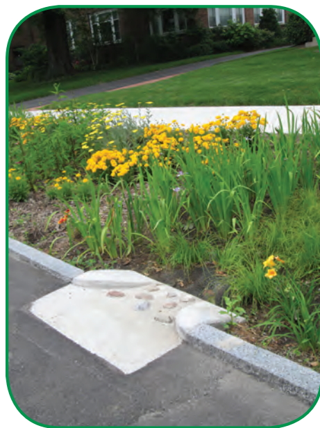
Energy dissipator between road and bioretention.
