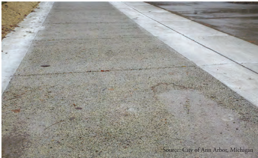
Completed permeable concrete alley.
