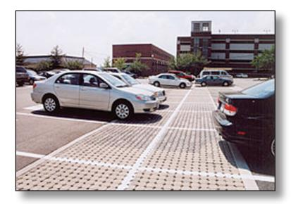
Figure 2.3.5a Reduced Parking Stalls with Permeable Paving Strips Photo Courtesy of: Washington, D.C. Navy
