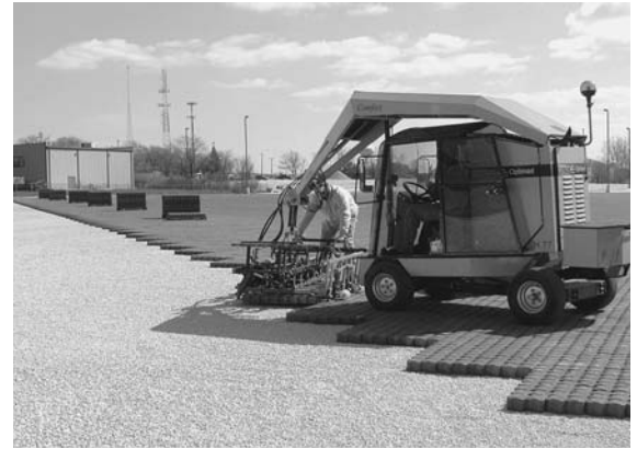
Mechanical Installation of Ecoloc® Permeable Pavers
