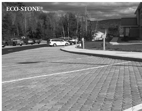
White Mountain National Forest Service Headquarters, NH
