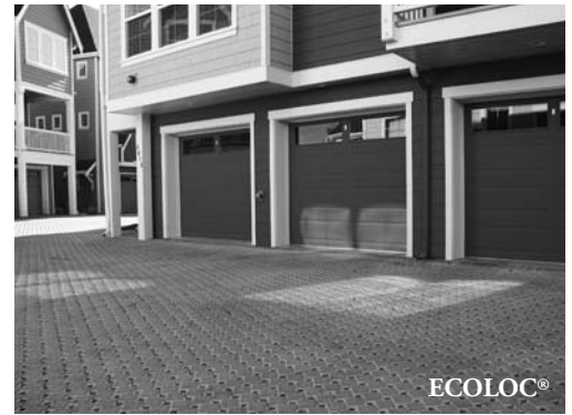
Highpoint Development, West Seattle, WA
