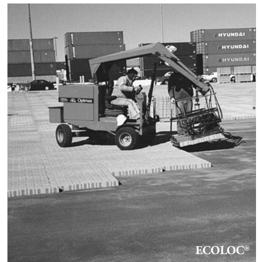
Howland Hook Marine Terminal Port of New York and New Jersey
