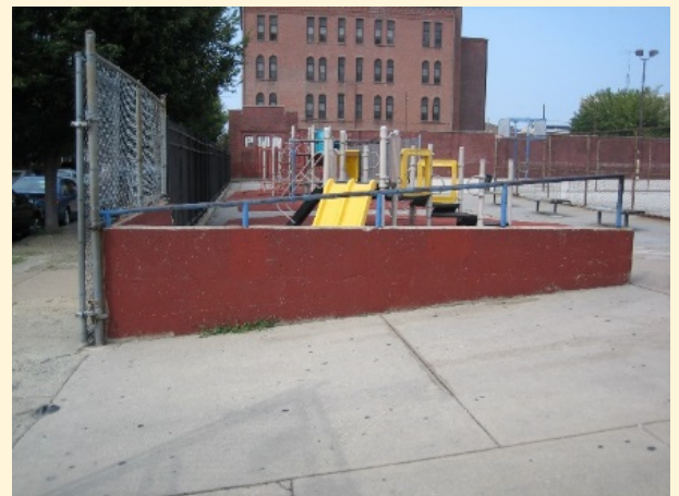
Figure 3. Top: east entrance of the park in 2011 after new green infrastructure elements were installed. Bottom: conditions in 2009, before renovation. (Source: Langan Engineering)
