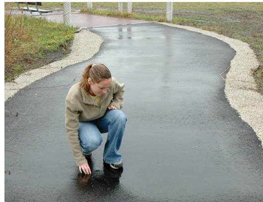
Figure 6: Permeable versus Conventional Asphalt
