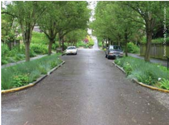
A pair of stormwater curb extensions installed along a low-density neighborhood street.
