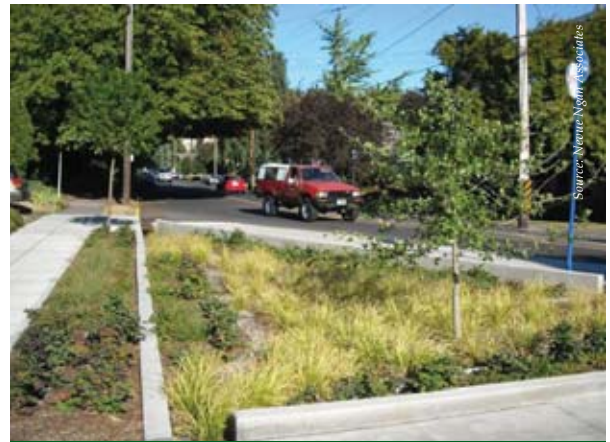
This large stormwater curb extension provides a safer intersection and enhanced bus stop.
