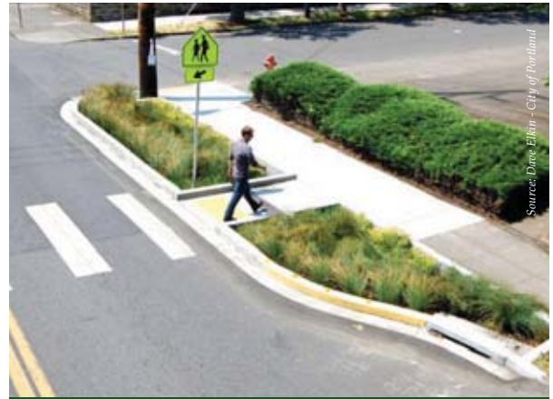
Accessible pedestrian ramps can also be integrated into the design of stormwater curb extensions.
