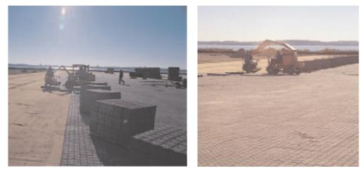
Like the past projects, recent construction of paving at Seagirt used mechanical equipment placing concrete pavers manufactured and stacked in the final laying pattern.
