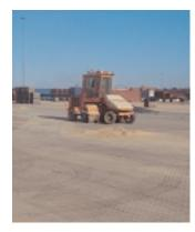
The contractor used a large sweeper to spread the fine sand into the joints between the millions of concrete pavers.
