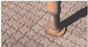
Truck trailer legs place point loads on the four year old interlocking concrete pavement with no damage in most areas.
